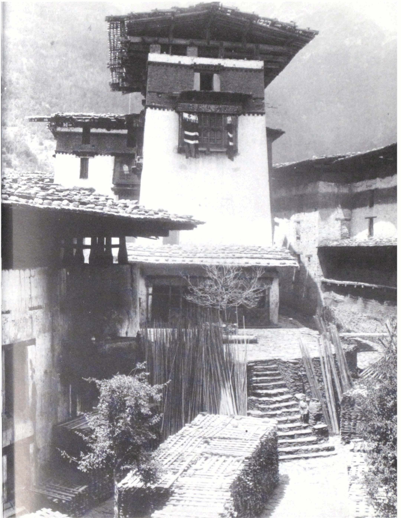
Interior courtyard of Drugyel Dzong with stacked wooden shingles ready for reroofing (White, 1905).
